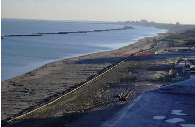
Figure 2.2. Picture of a long pipeline during a nourishment at Lido degli Scacchi
