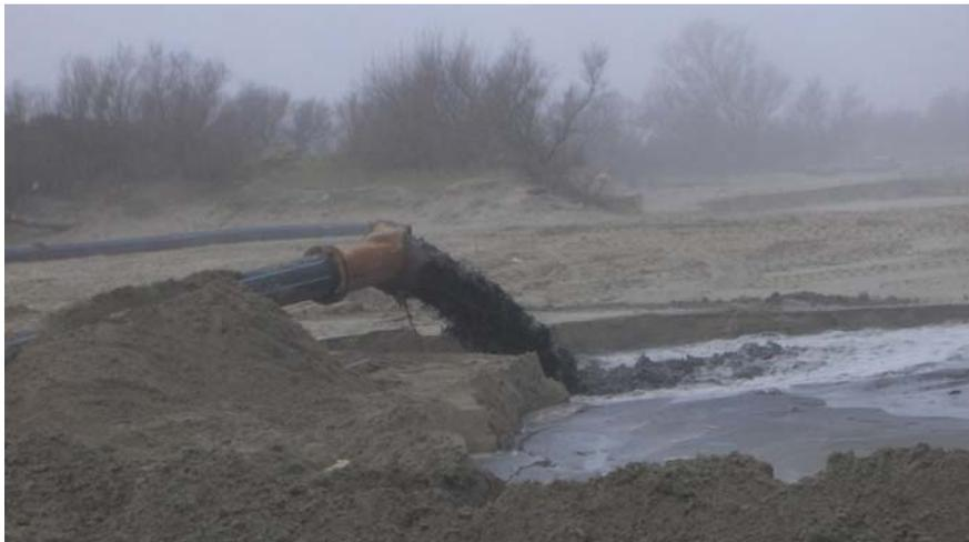
Figure 2.3. A pipeline delivering diluted sand precisely where it is needed
