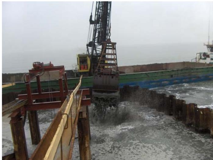
*Figure 2.6. Deposition of sand into from the barge into the delimited area*
